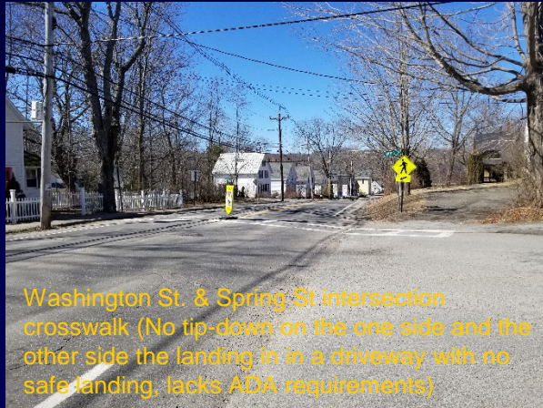
Washington St. & Trim St intersection crosswalk (No tip-down on the one side and the other side has no safe landing, lacks ADA requirements)
